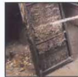
Trapped debris is hosed away
